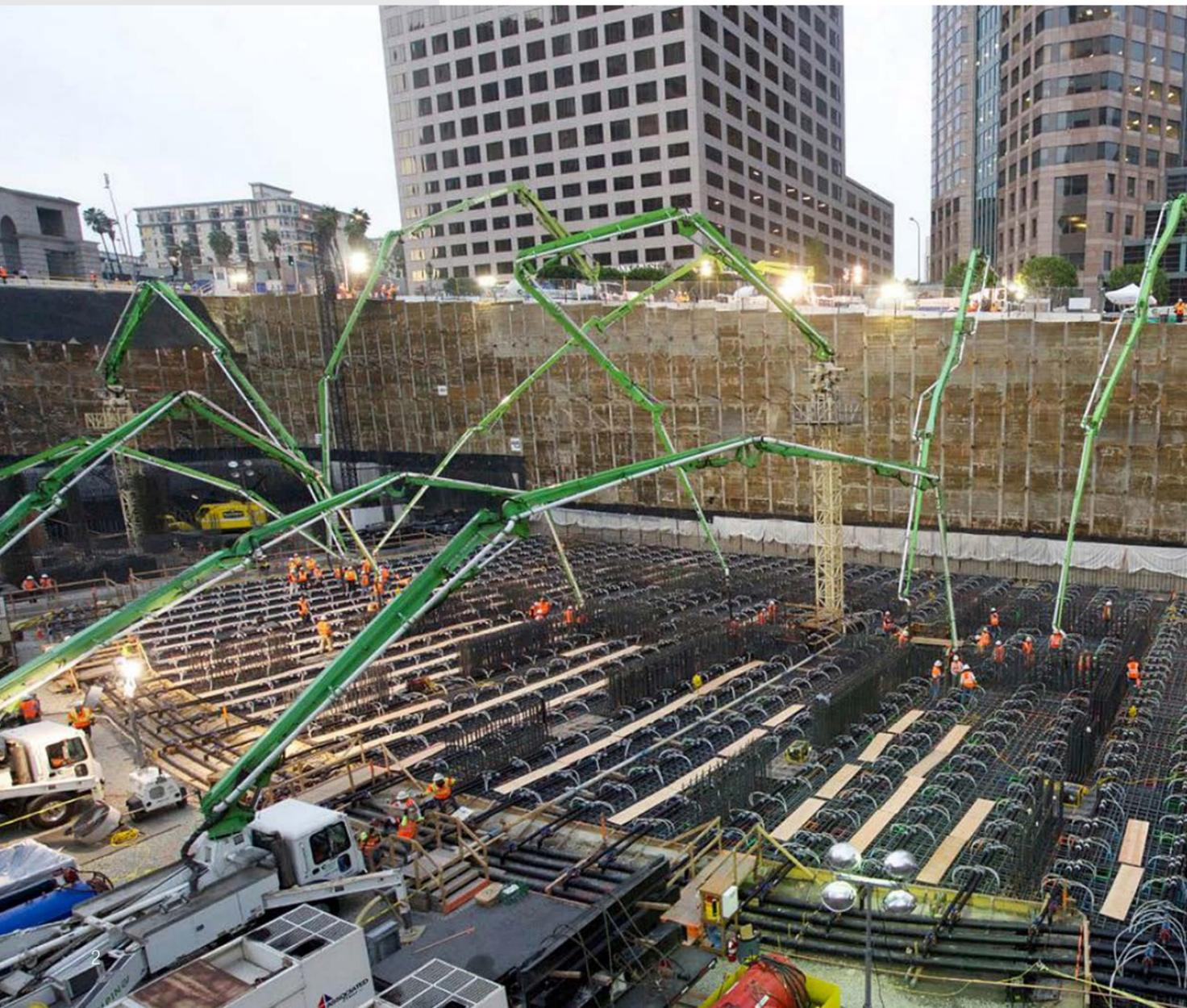
**Truck-mounted concrete pumps**
